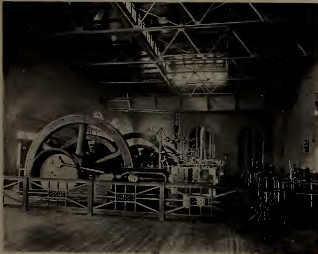
ENGINE-ROOM POWER PLANT PORTLAND RAILROAD COMPANY, Portland, Me. Sheaff & Jaastad, Engineers, 85 Water Street, Boston.
